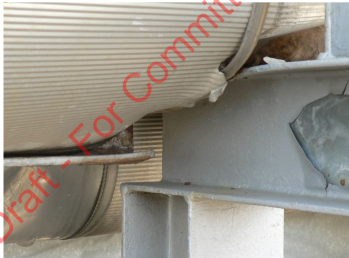
Figure 18: Insulation Jacket Remove and Repair
