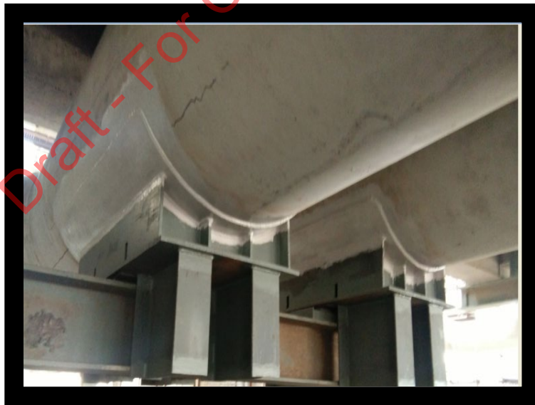
Figure 9: Welded Pipe Saddle
