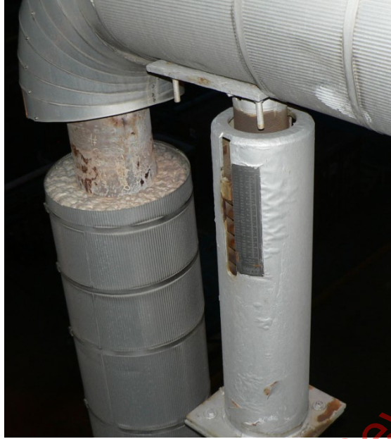
Figure 19: Insulation Remove and Repair
