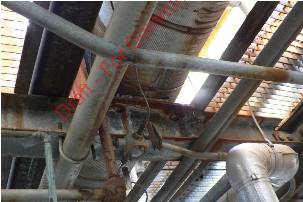
Figure 20: Difficult Access for all NDT Methods
